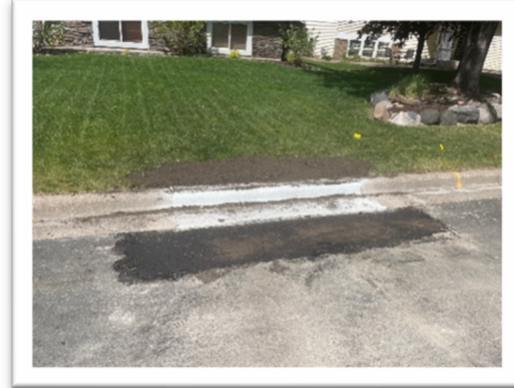
Above Center: Backfilling curb & gutter with top soil
