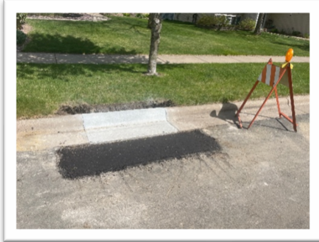
Above Left: Bituminous patching of curb & gutter
