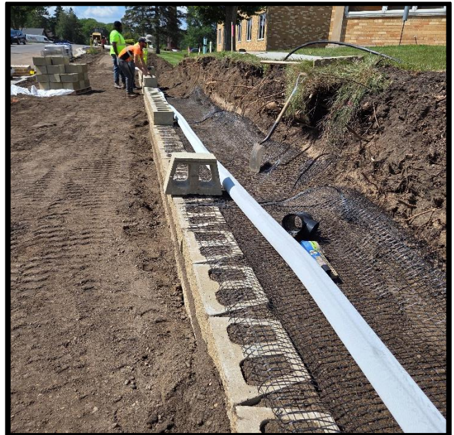
Installation of retaining walls
