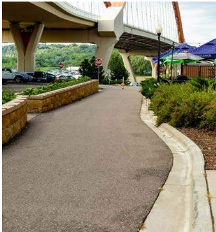
Trail access at the Hwy 61 bridge
