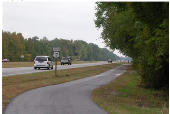
Off-road paved trail along divided highway
