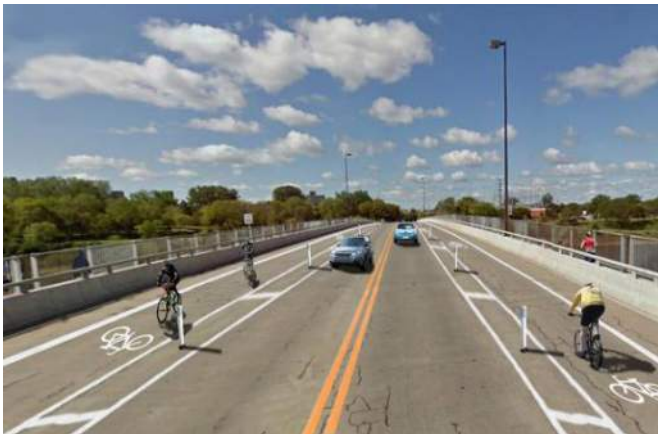
Protected bike lanes on bridge with plastic bollards and separate side path for pedestrians
