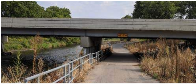
Trail underpass of Hwy 47/Vermillion Road
