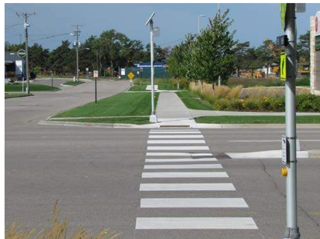
Marked crosswalk with HAWK signal
