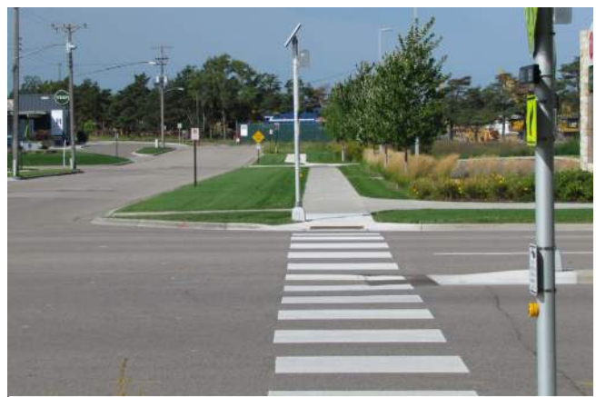
Marked crosswalk with HAWK signal
