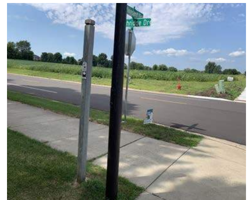
Although there is a 10-mile route marker at the intersection of Northridge Drive and Pleasant Drive on the 10-mile loop, it is unclear that the wide sidewalk functions as a multi-use trail. More visible directional signage and pavement markings would help provide legibility to the trail route.
