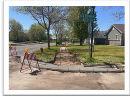
Above Right: New Curb at Pedestrian Ramp
