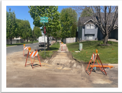
Above Left: Removal of Pedestrian Ramp
