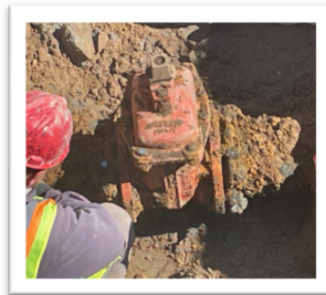
Above Center: Rebolting of Gate Valve
