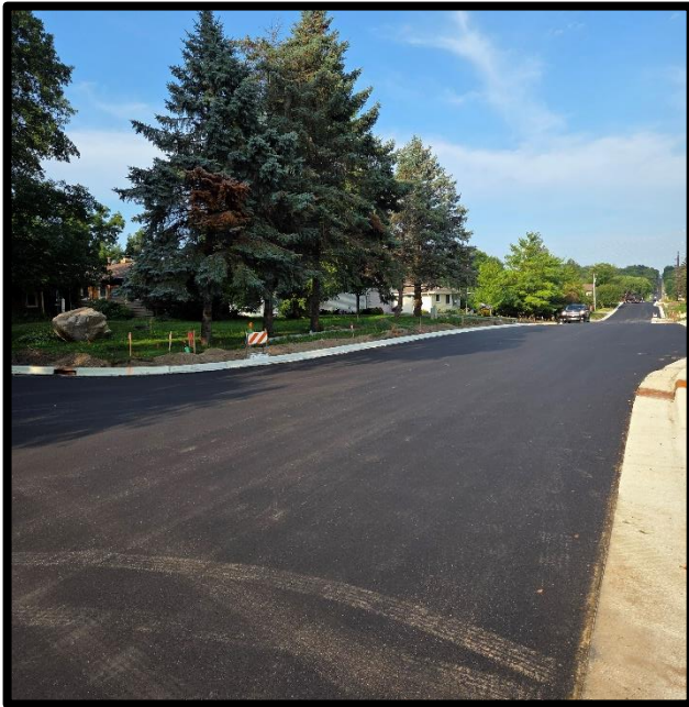
Completed paving of the first layer on 1 st Street
