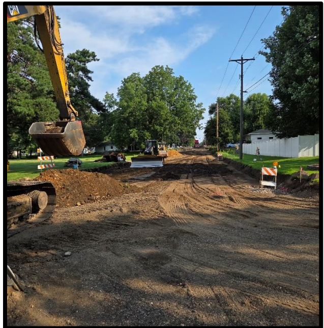
Grading of road base
