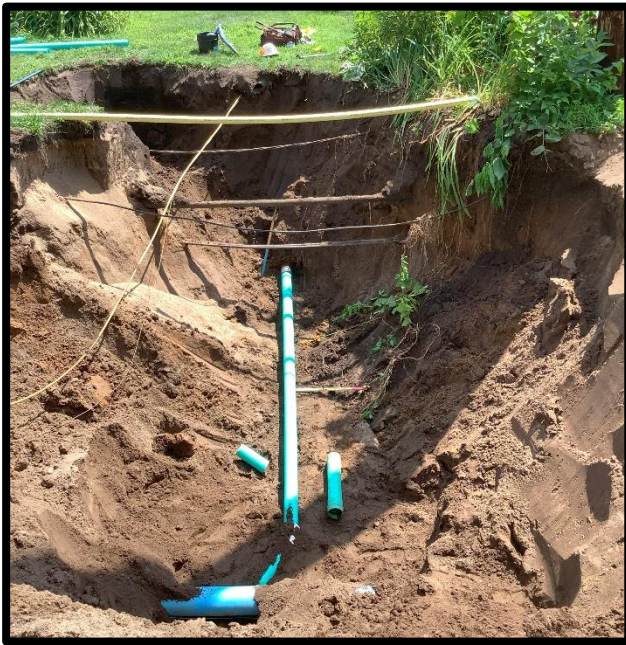
Sanitary sewer service replacement
