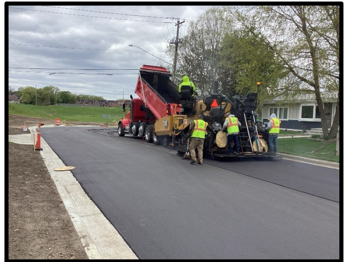
Paving 7 th Street
