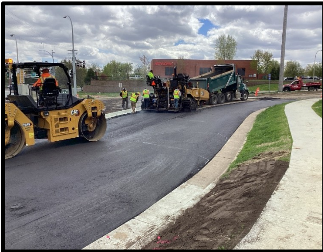
Paving North Frontage Road
