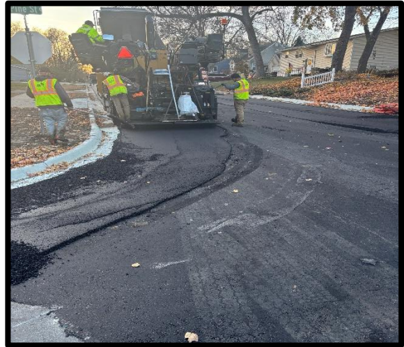
Installing Temporary Asphalt Wedge
