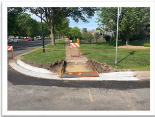
Left: Preparing pedestrian ramp for concrete
