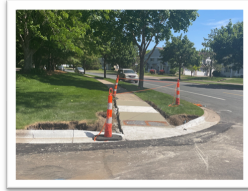
Right: Pedestrian ramp poured
