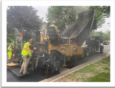
Photo: Paving Street
