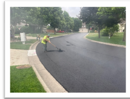
Photo: Raking Blacktop Mix Around Manhole
