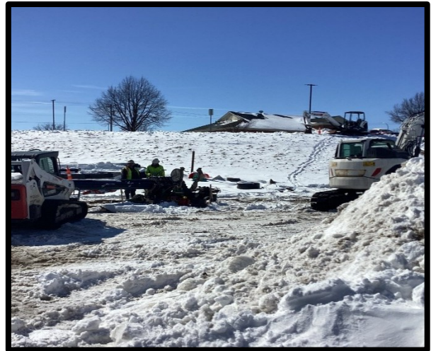
Fusing Watermain Pipe
