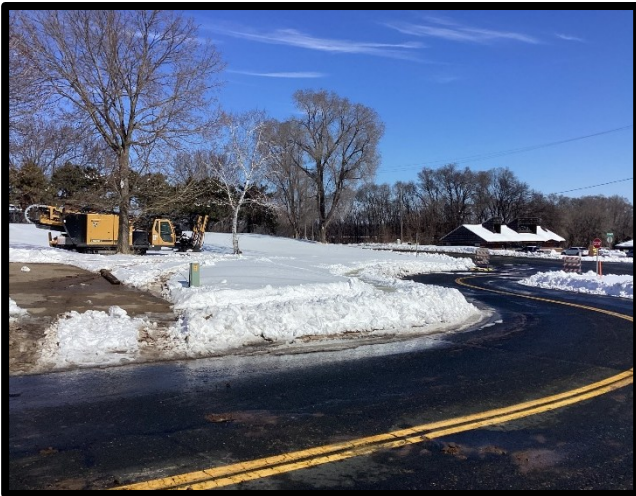
Setting up the Directional Drill Rig
