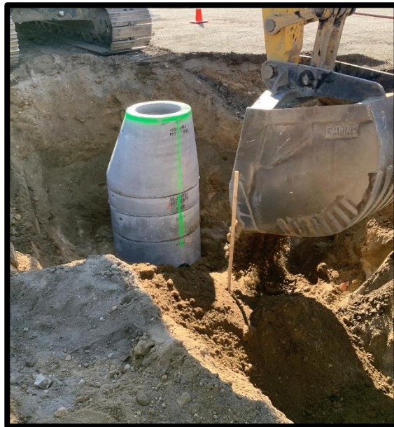
Sanitary sewer improvements
