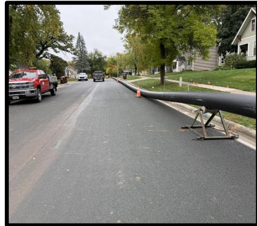
Fusing Watermain Pipe
