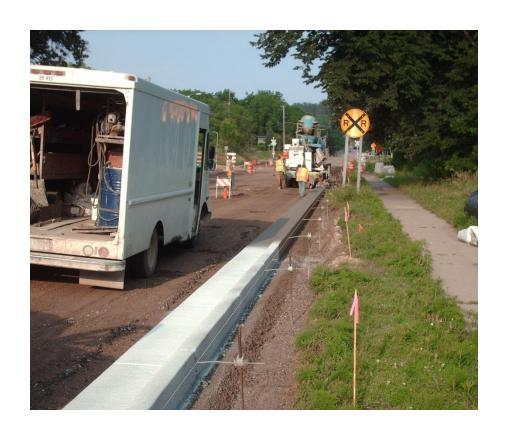
After the gravel base has been prepared, concrete curb and gutter is installed. Access by vehicles to driveways is not permitted for 7 days after all concrete has been placed to allow for this material to build adequate strength. Parking in front of homes during the evenings is allowed.
