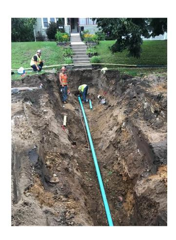
Sanitary sewer mains and services are lined or replaced with new, high strength, longer lasting materials. Deep trenches are often required, which can limit access to residences for parts of the day.
