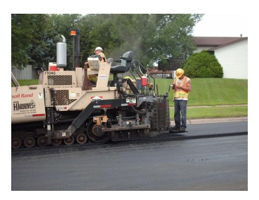
All other major construction tasks have been completed. This leaves only the placement of the final (wearing) course of asphalt pavement. Afterward, the street and utility improvements are then considered substantially complete.
