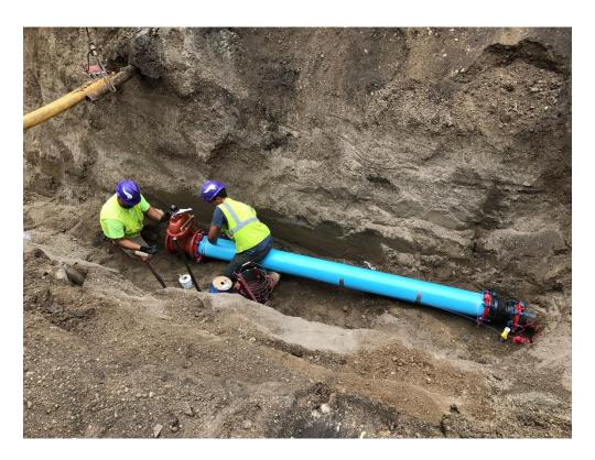
Defective and aging parts of the existing water system are removed and replaced. These components include valves, fire hydrants, main lines, and service pipes and connections. The water system is typically placed closer to the surface than the sanitary sewer system, but also requires deep trenching. This activity normally takes place after sanitary sewer work is completed.
