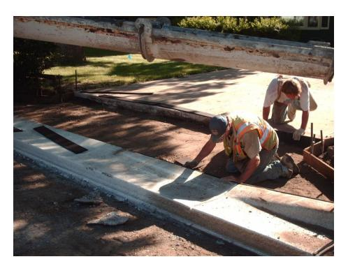
Concrete aprons are installed for some driveways. If any portion of the driveway is left to be filled in, it is replaced with the same material (asphalt, concrete, or gravel) as the existing driveway. This step sometimes occurs after the curb has been placed but before any asphalt paving.
