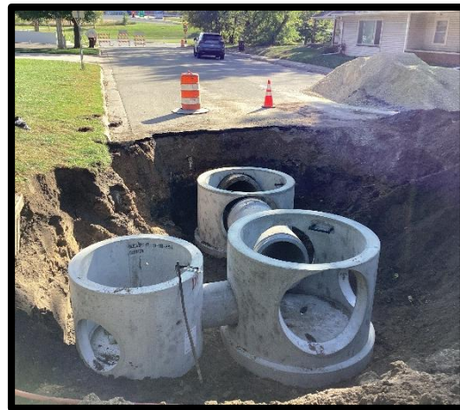
Storm Sewer Installation
