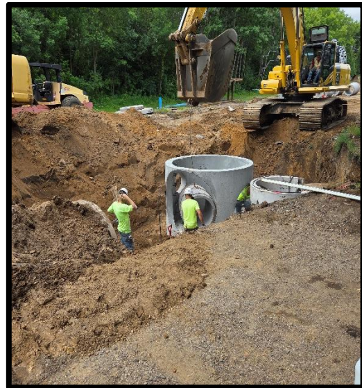
Storm sewer improvements
