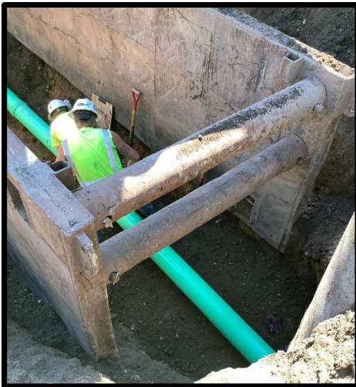
Sanitary sewer improvements
