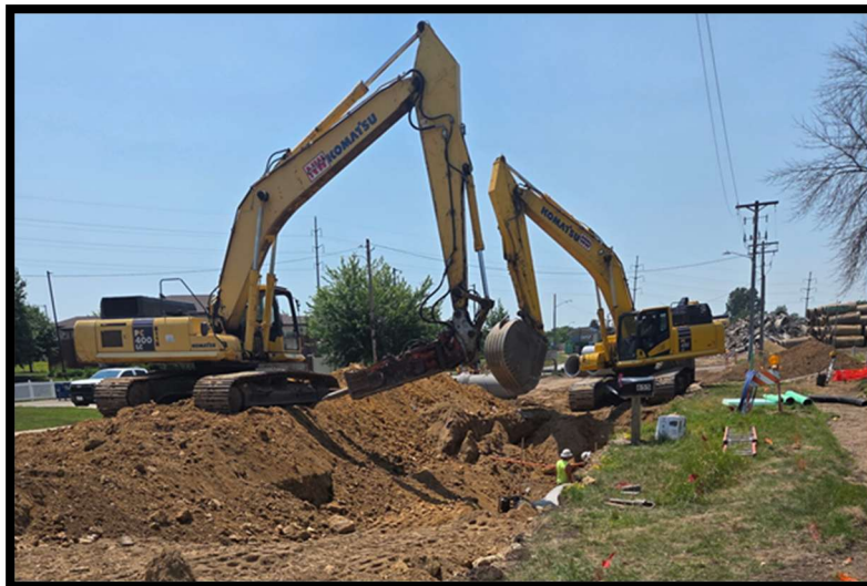
Excavation for Storm Sewer Improvements
