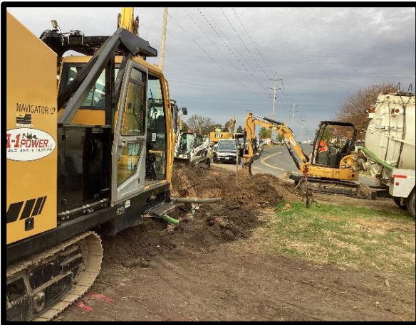
Directional Drilling Watermain on North Frontage Rd
