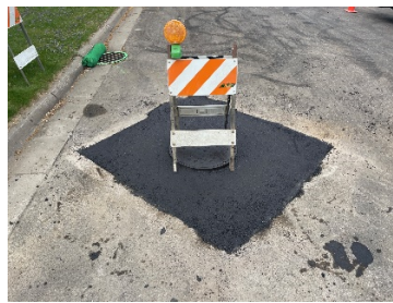
Above Center: Bituminous patching
