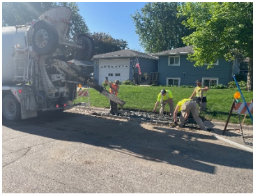
Above Left: Pouring curb and gutter
