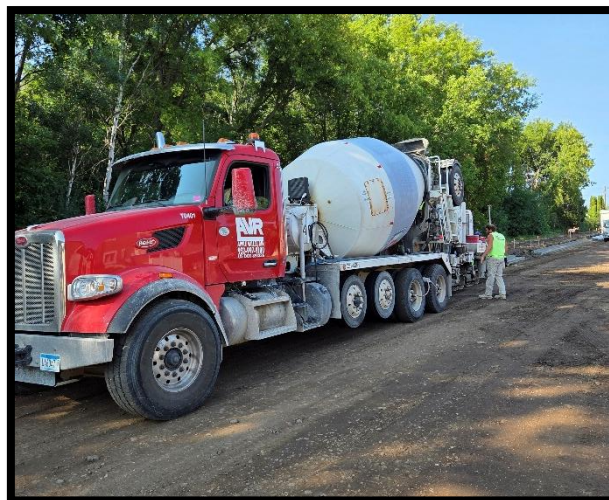
Concrete curb and gutter being installed
