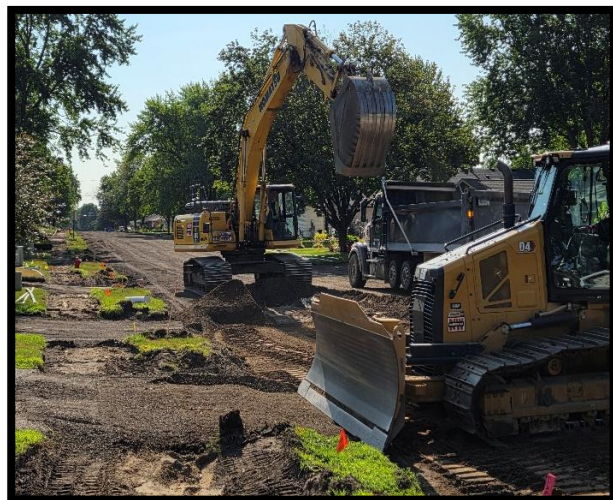
Street removals along 4 th Street
