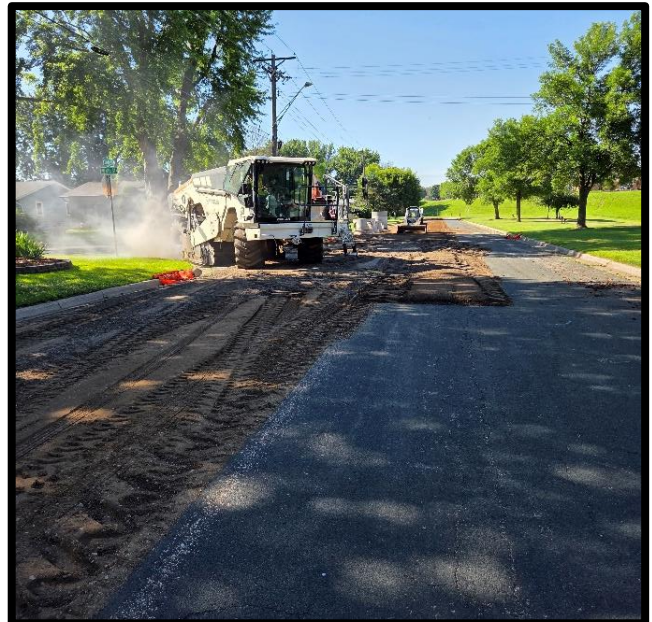
Reclaiming (grinding) of existing asphalt
