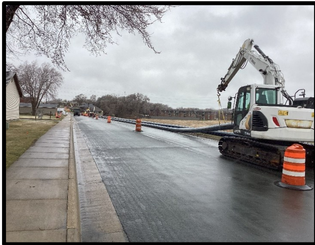
Watermain Pipe Being Pulled into Bore Hole
