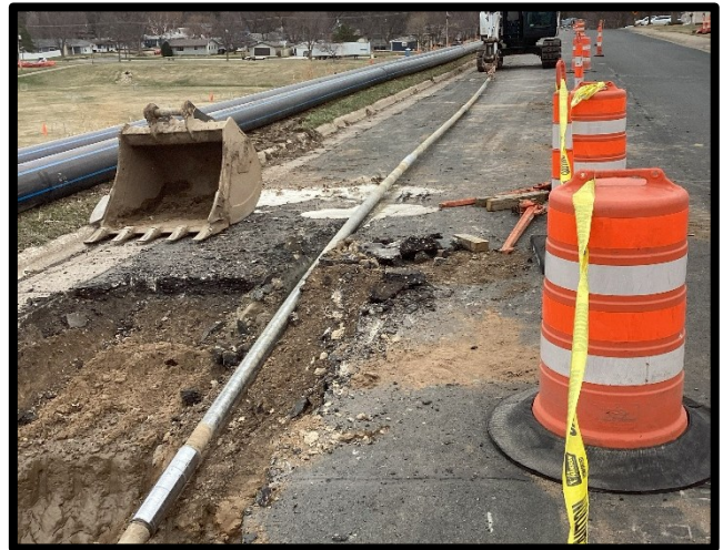
Drill Rod Existing the Bore Hole / Preparing for Pipe Tie On
