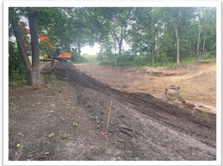
Photo: Excavation of Pond
