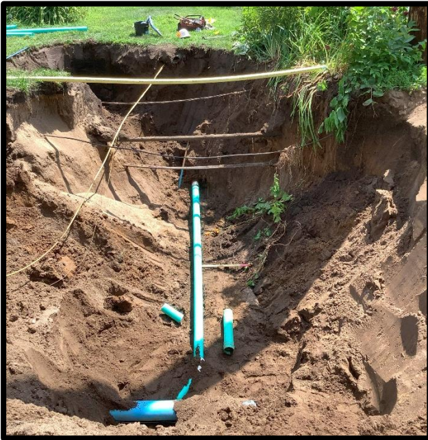
Sanitary sewer service replacements
