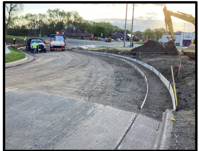
Setting Forms for Curb Replacement
