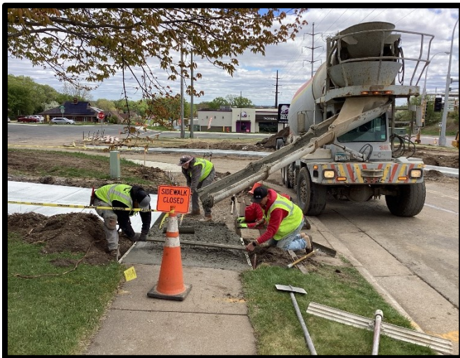
Replacing Concrete Sidewalk
