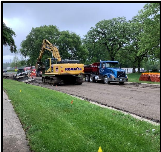
Removing existing concrete curb and gutter
