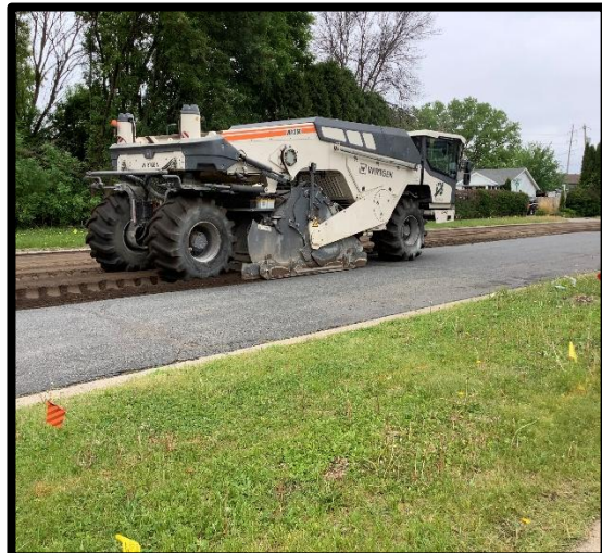
Reclaiming (grinding) of existing pavement
