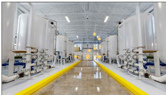
GAC treatment vessels to remove PFAS
