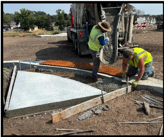
Concrete Pedestrian Ramp Installation
