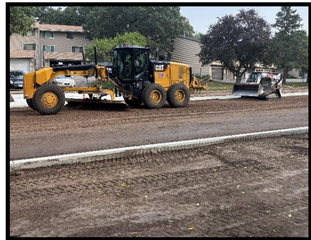
Grading of road base in preparation for asphalt
