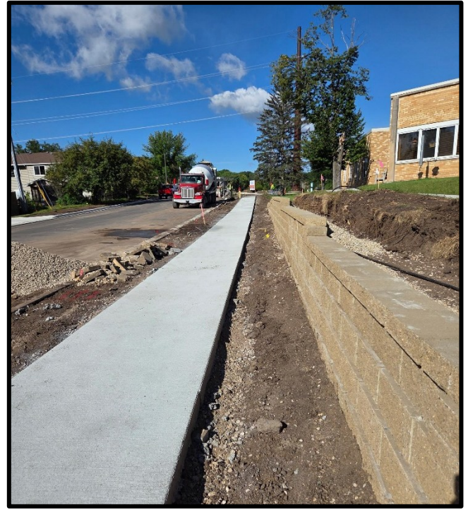
Concrete sidewalk and retaining wall installation on 1 st Street
