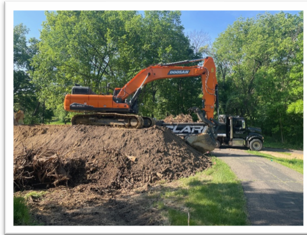
Above: Excavating pond and hauling out excess soil.
