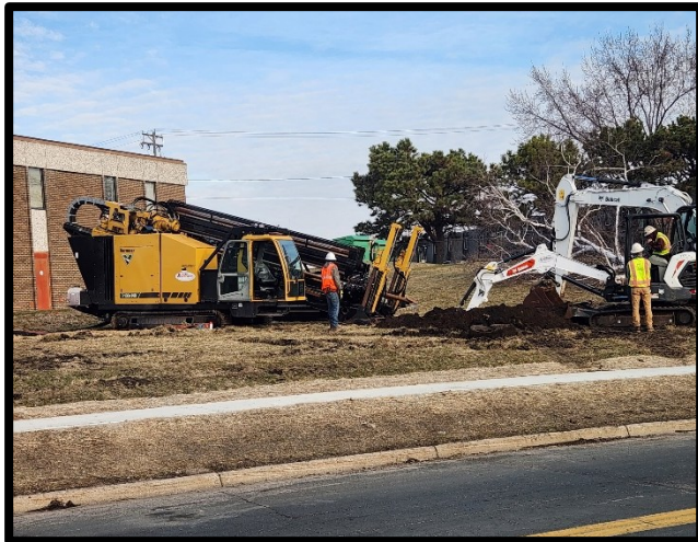
Horizontal Directional Drilling the Bore Hole
