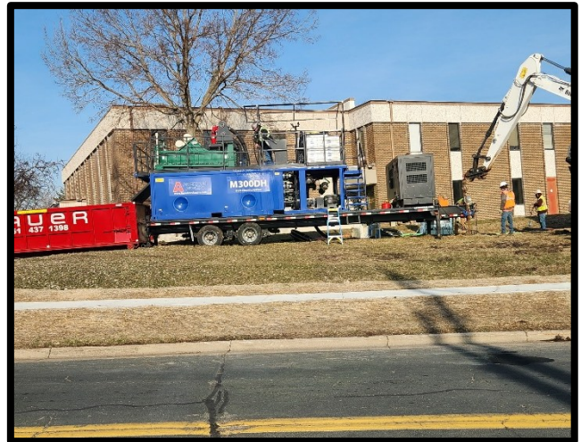
HDD Mixing/Pumping Unit to Circulate Drilling Fluid/Mud
