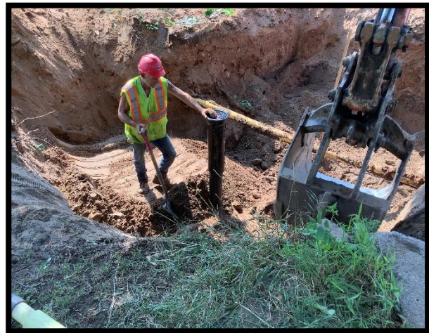
Watermain improvements on 4 th Street
