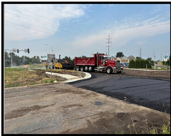
Paving of Pleasant Drive
