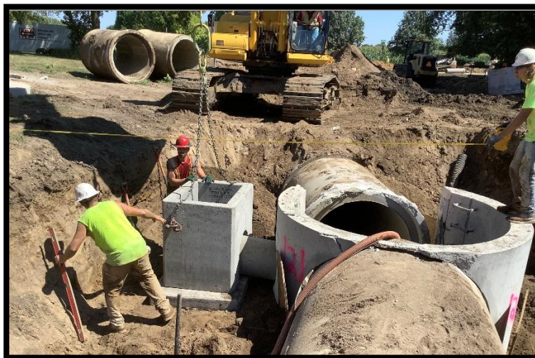
Excavation for Storm Sewer Improvements
