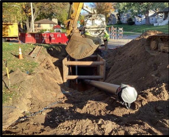
Pulling Watermain Pipe In Place
