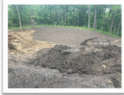
Above (all): Excavating ponding basin
