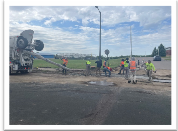
Above: Pouring concrete pedestrian ramp on 4 th St
