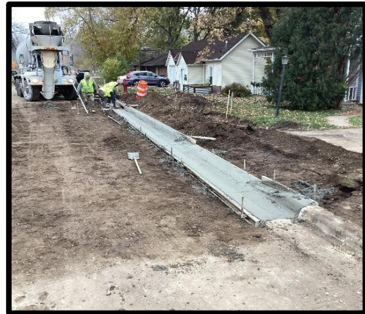
Installing Concrete Curb
