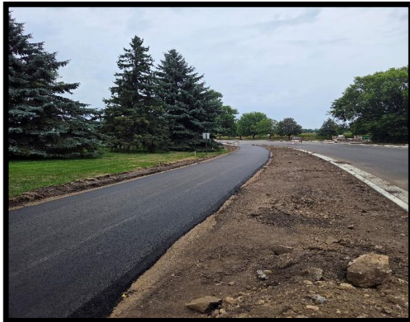
Completed trail paving along Pleasant Drive
