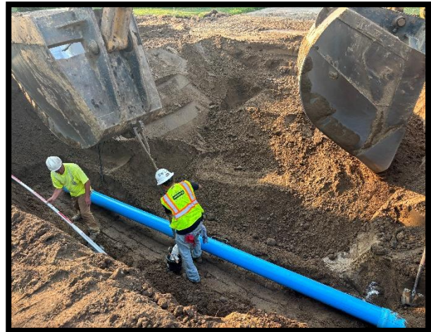
Watermain improvements on 4 th Street
