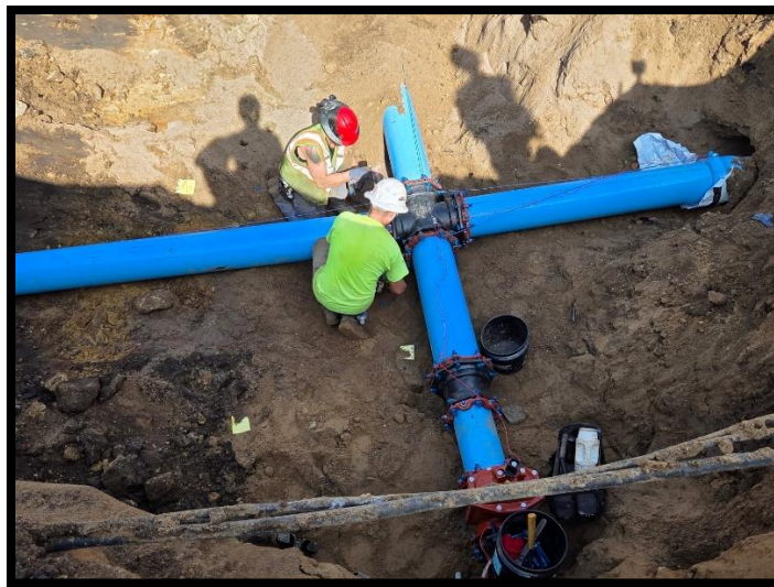
New watermain crossing installation
