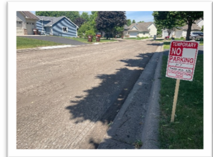
Right: Milling Complete
