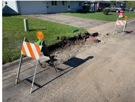
Above Center: Curb Removed
