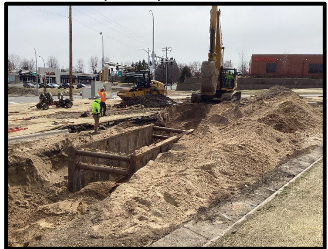
Installing Watermain Crossing N. Frontage at Westview
