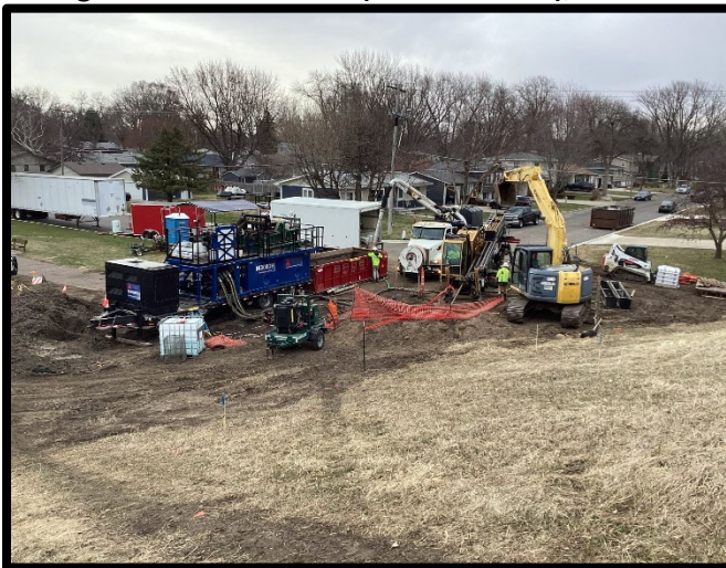
Drilling Watermain from Lions Park to Mid-block N Frontage
