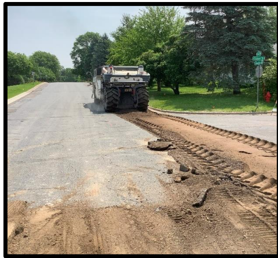
Reclaiming (grinding) of existing pavement
