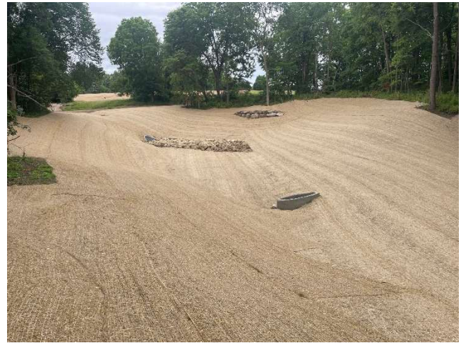
Right Photo: Basin Restored
