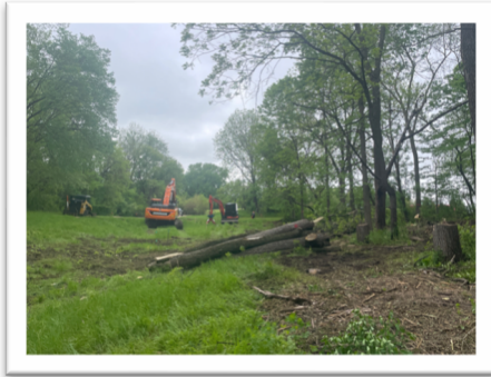
Above Left: Tree Removal
