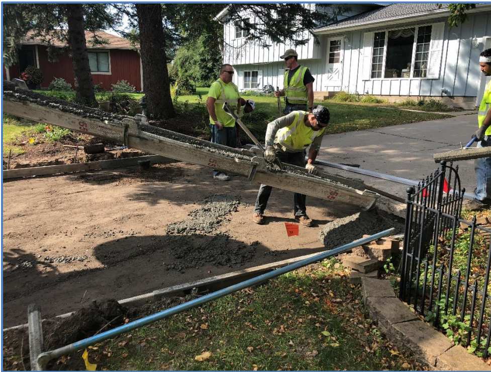
Pouring a concrete driveway on Manor Ct
