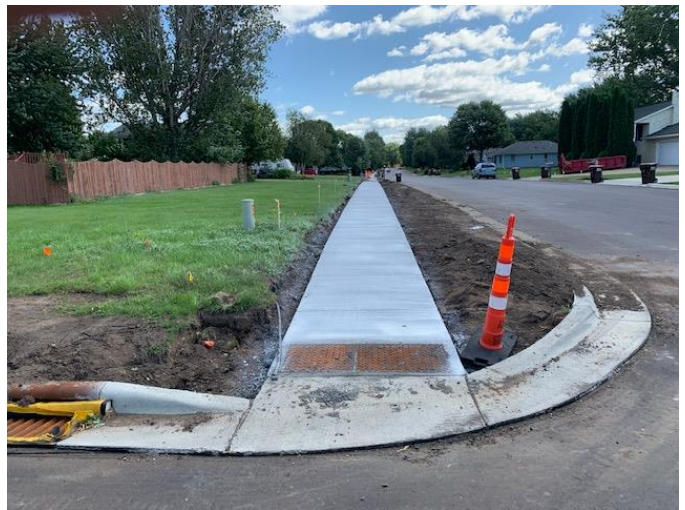
Newly installed sidewalk on 31 st St
