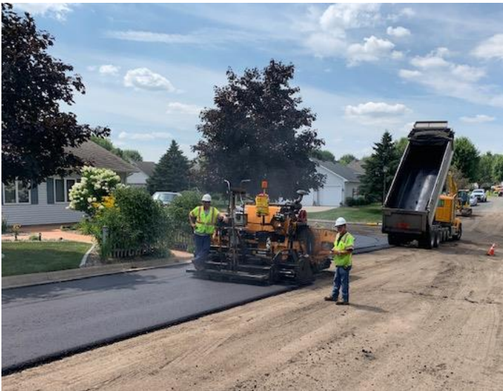
Paving in progress on South Park Court
