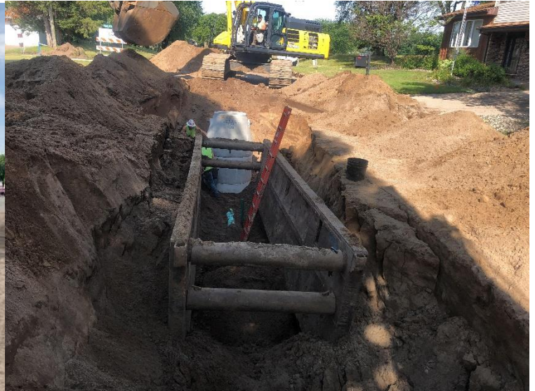
A new sanitary sewer manhole is installed in 19 th Street
