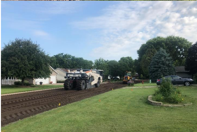
Clockwise from top left: Grading on Edgewood Ln in preparation for placement of gravel base. A new sanitary sewer service is installed beneath the new water main on 21 st St. Reclamation in progress on Highview Knoll. Sanitary sewer lining on 21 st Street.
