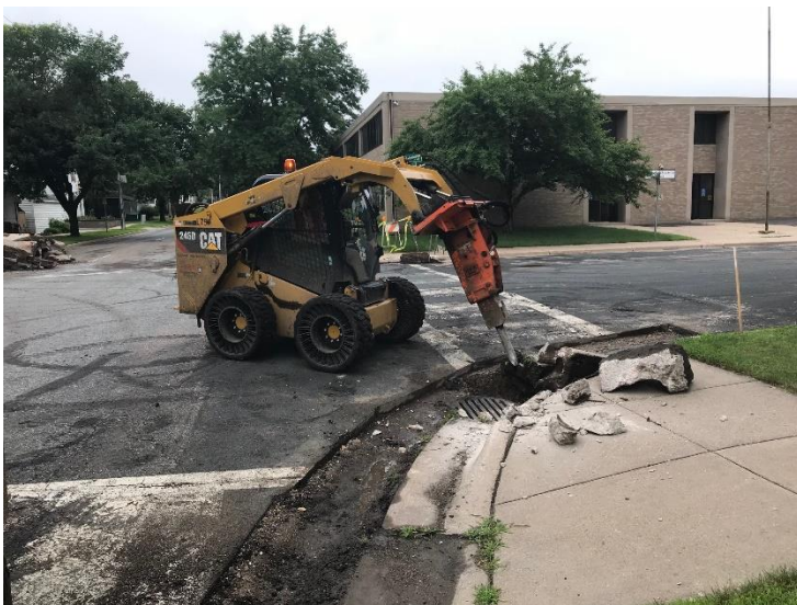
Example of removals for spot curb replacement
